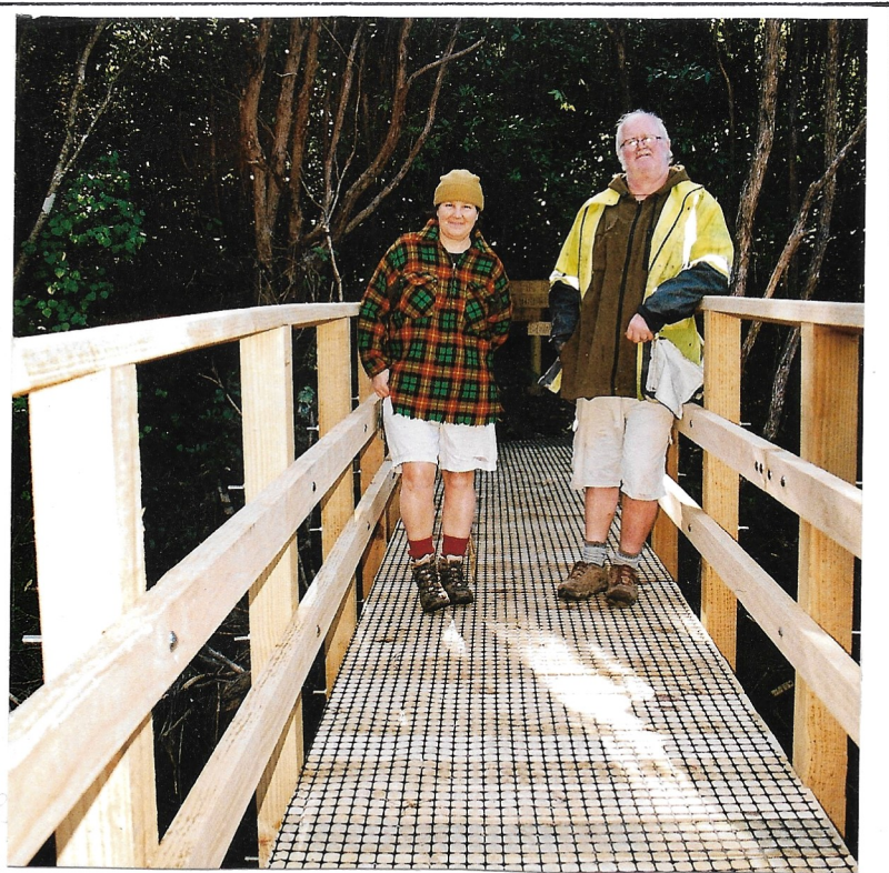
Engineer Kate Zwartz and Bridge Builder Paul Newport on the completed bridge across Narbey Stream. 22 Aug.
